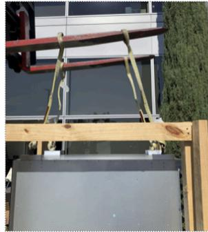
4. Place the chassis on the transport lift (Server Lift SL-1000X® Super-Duty Lift) with the lift platen in the neutral position and the chassis aligned for moving into the rack.
